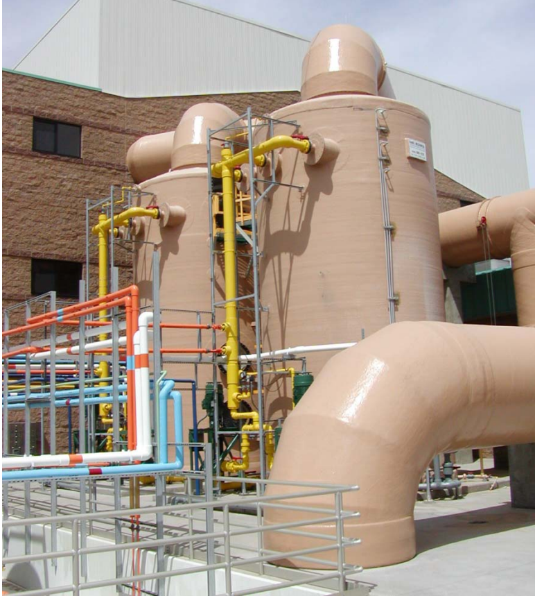
Picture #3: City of Mesa Northwest WRP, Arizona (60,000 CFM)
