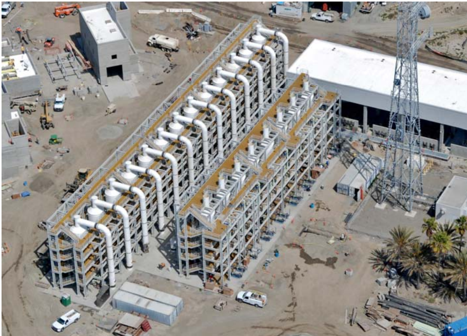
Orange County Sanitation District, Huntington Beach, California (180,000 CFM)
